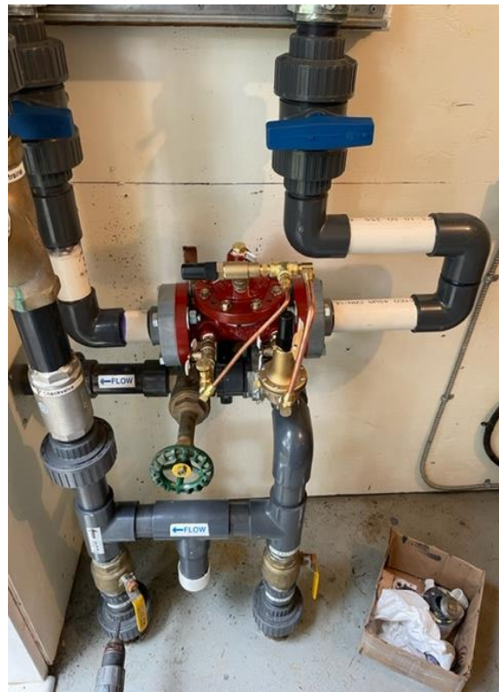
New PRV installed and fully operational.
