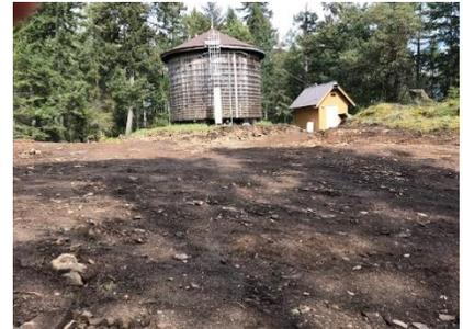
If you tour the water tank site you will notice some changes. A number of trees have been removed, the site has been graded and the power and telephone cables have been moved out of the planned construction area.
